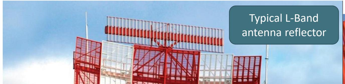
Typical L-Band antenna reflector
