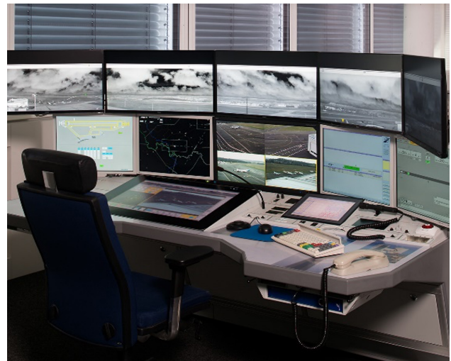
Figure Case Study 4: Controller Working Position in Leipzig Centre
